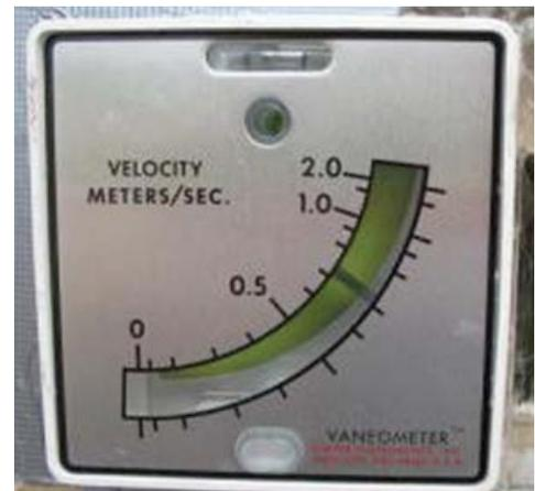
**Figure 4** Example of a 'swinging vane' fitted to a spray room
