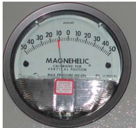
**Figure 3** Example of a manometer fitted to a spray booth
